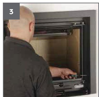
With a frame with finish, adjust the depth so that it is fitted correctly [pic. 3]. In the case of a thin frame, screw in the two M5 screws in the centre of top horizontal part [pic. 4].
