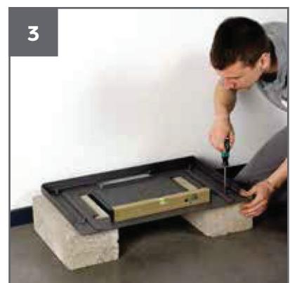
4 headless M10 screws (supplied with the fireplace) can be used to level the plate [photo 3]. Remember to take out the flexible tube for the convection air.
